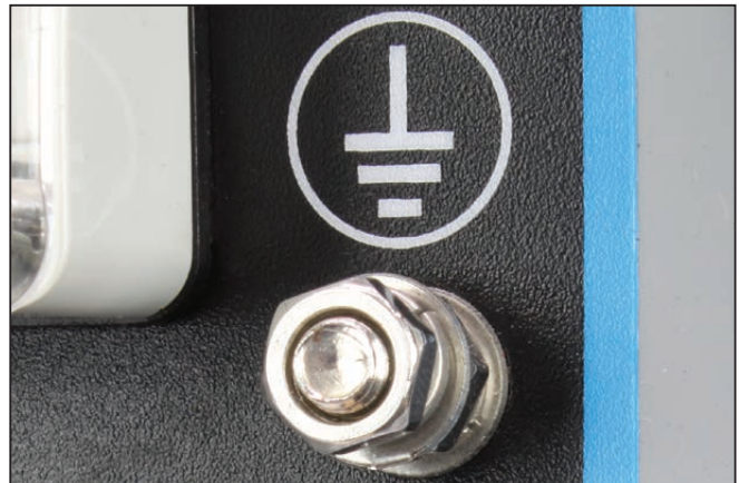
Figure 12 – Frame Terminal on the Control Panel
