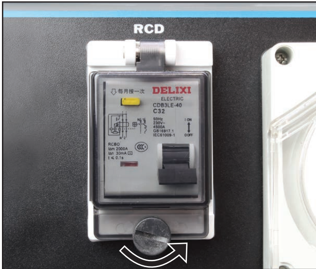
Figure 50 – Opening the RCD Safety Switch Cover
